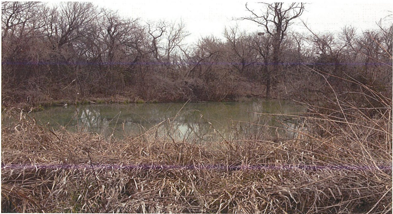
Figure 14: Standing Water at Toe of Dam
