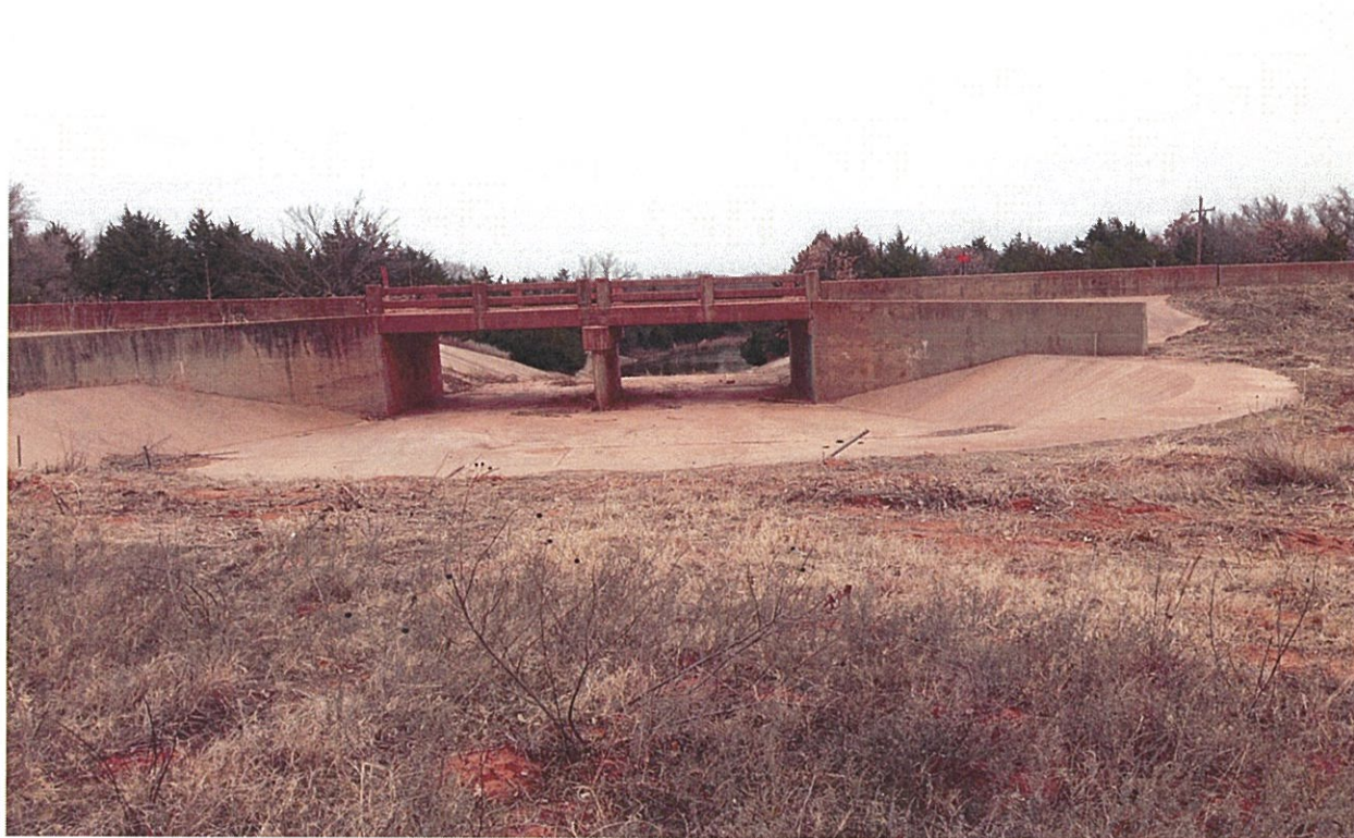
Figure 245: West Spillway – Photo Facing N
