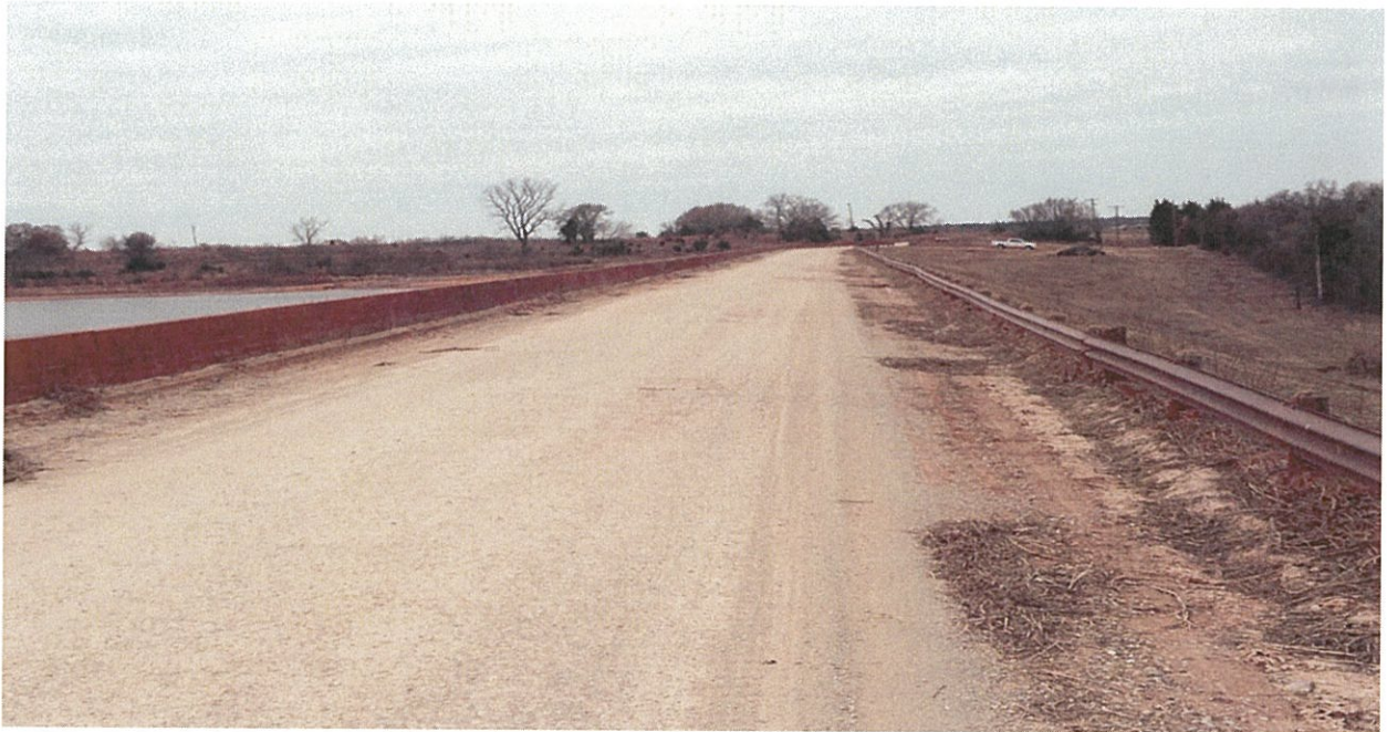
Figure 9: Crest of Dam – Photo Facing West
