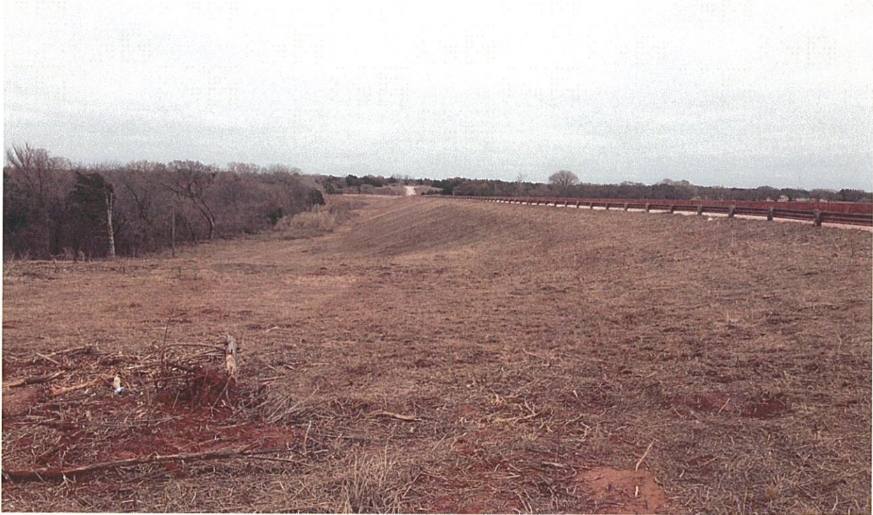
Figure 11: Downstream Slope - Facing East
