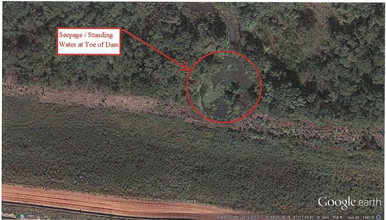
Figure 17: Aerial Image of Seepage at Toe
