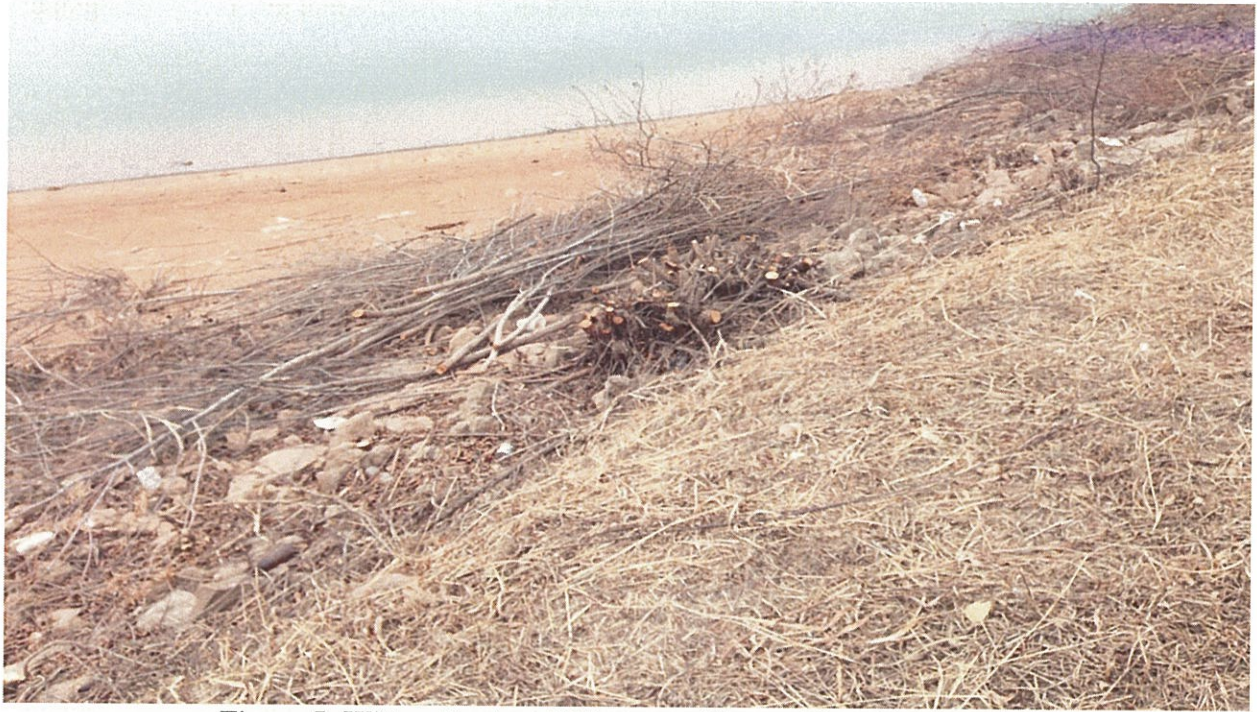
Figure 5: Willow Root on E Upstream Slope – Photo Facing SSW
