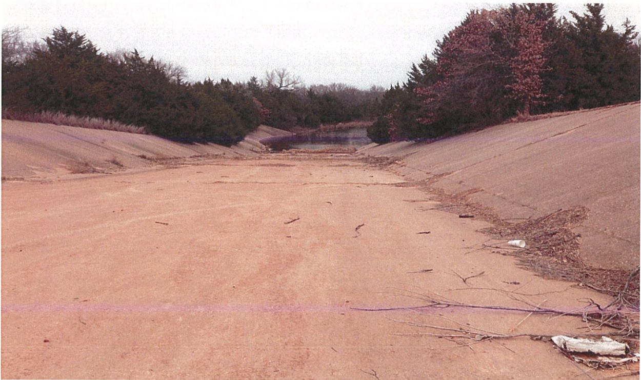
Figure 267: West Spillway Channel
