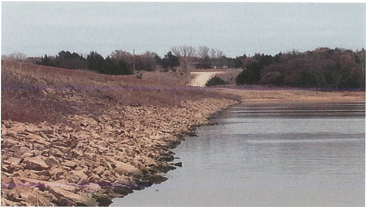
Figure 2: Upstream Slope of Dam – Photo Facing ENE
