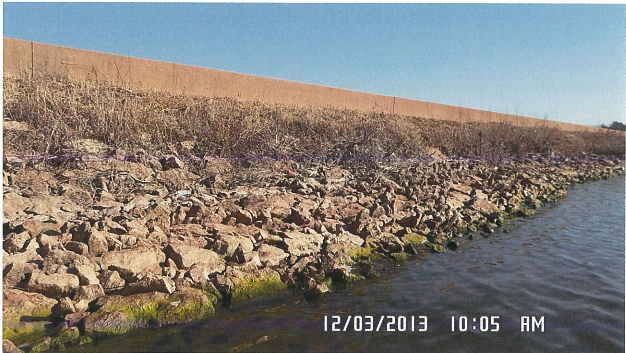
Figure 4: West End of Upstream Slope – Photo Facing NE
