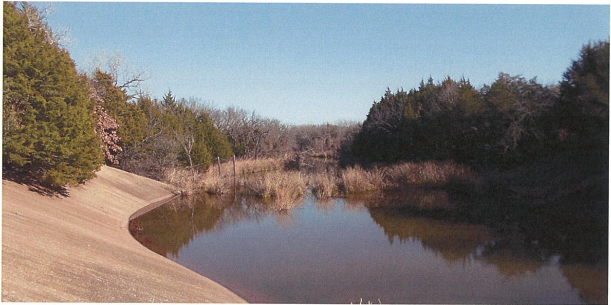
Figure 32: Stilling Basin - Photo Facing NNE
