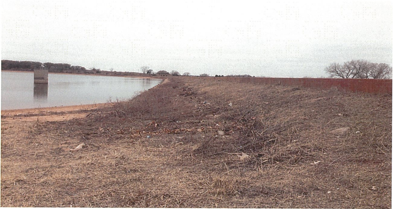
Figure 1: Upstream Slope of Dam – Photo Facing WNW
