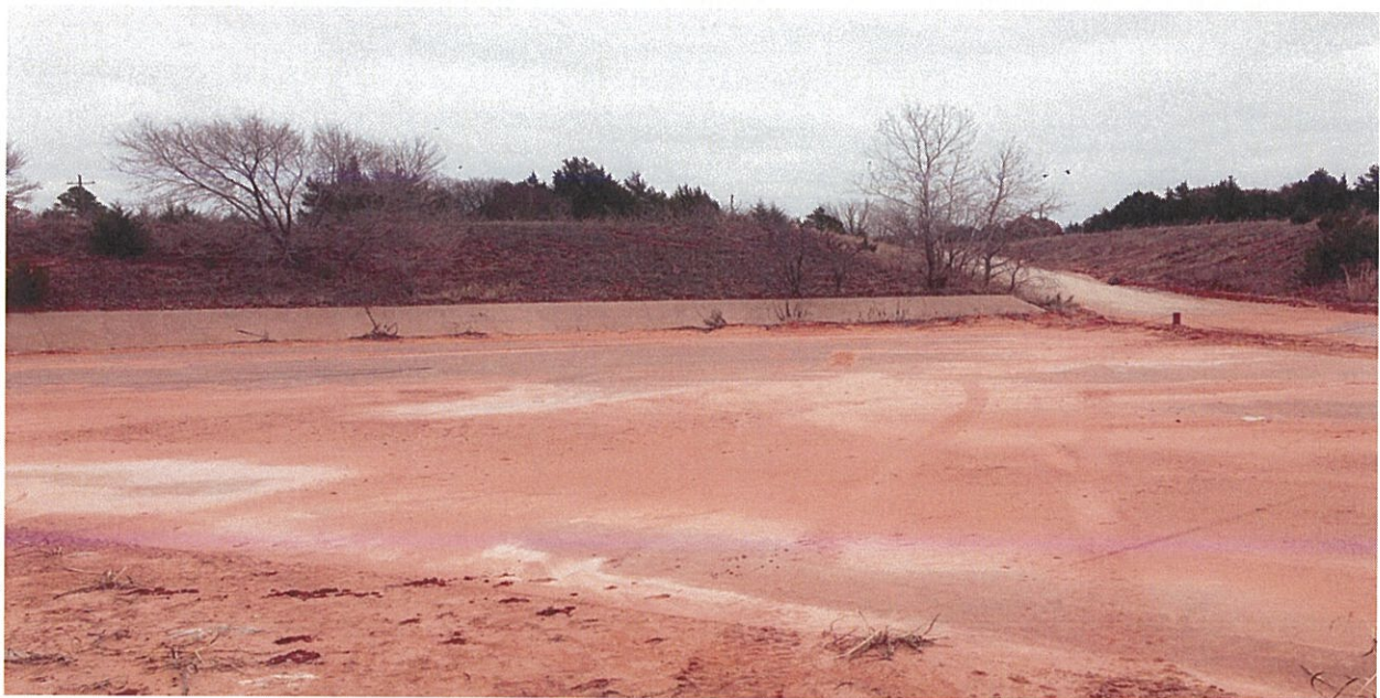
Figure 29: Emergency (East) Spillway - Photo Facing E
