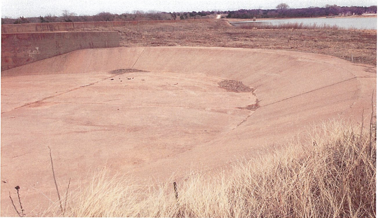
Figure 256: West Spillway – Photo Facing E
