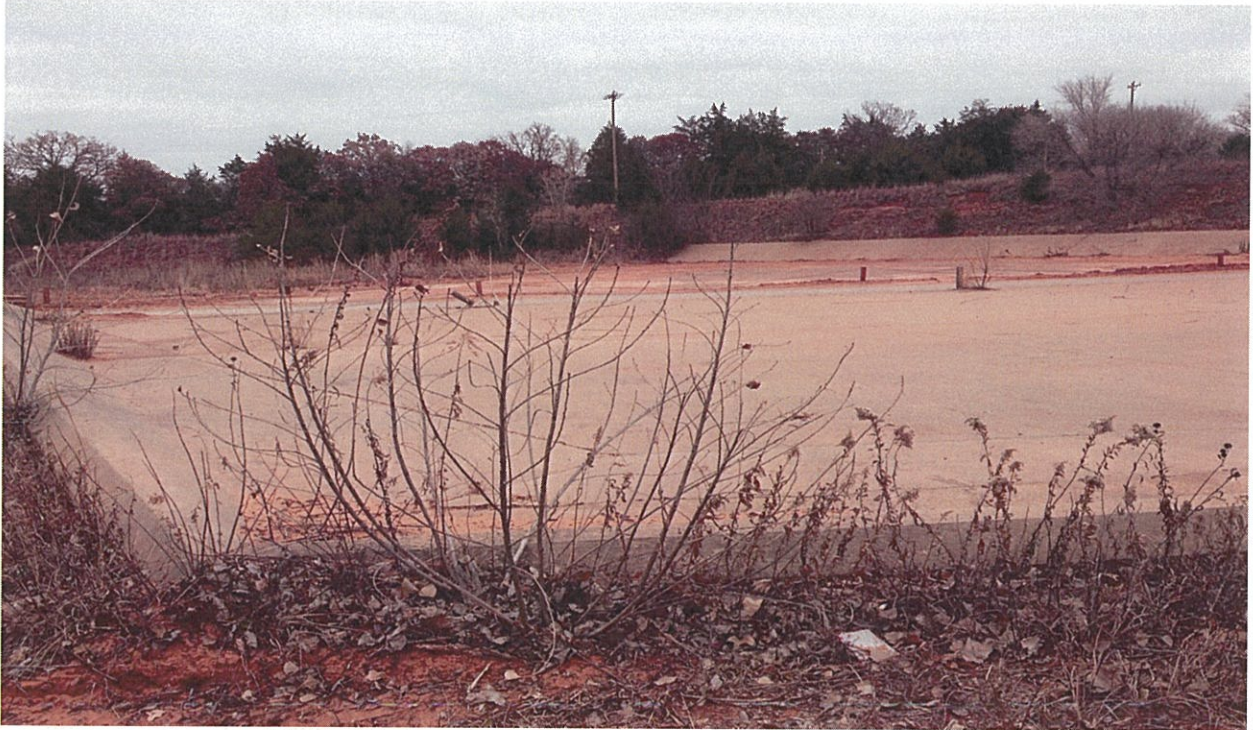
Figure 30: Emergency (East) Spillway - Photo Facing NE
