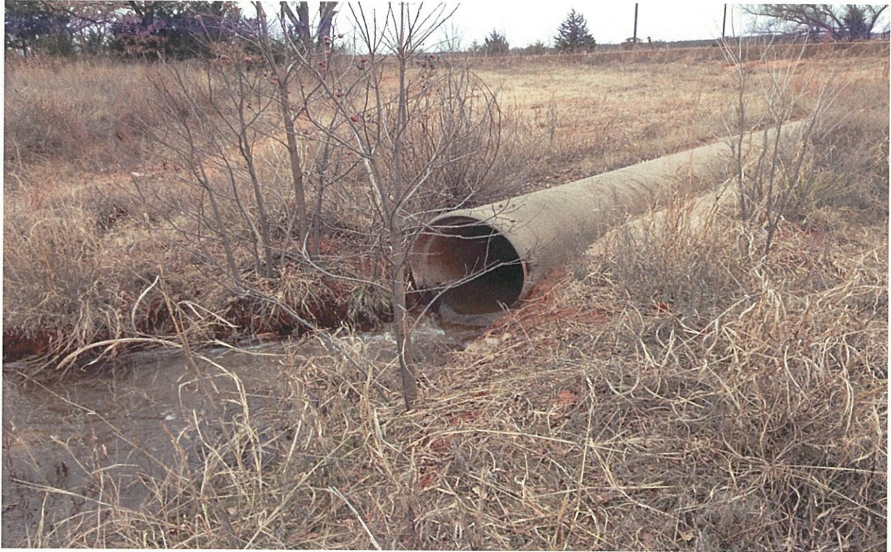
Figure 7: Cottonwood Creek Influent Pipe West End of Upstream Slope
