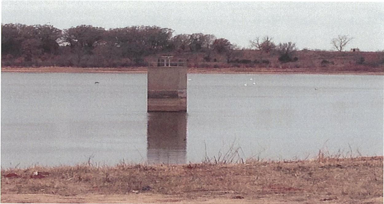
Figure 21: Inlet Structure – Photo Facing SW
