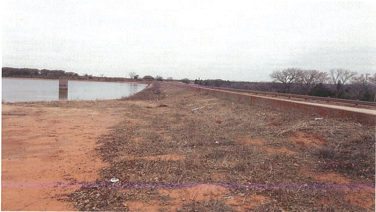
Figure 6: East Abutment– Photo Facing ENE
