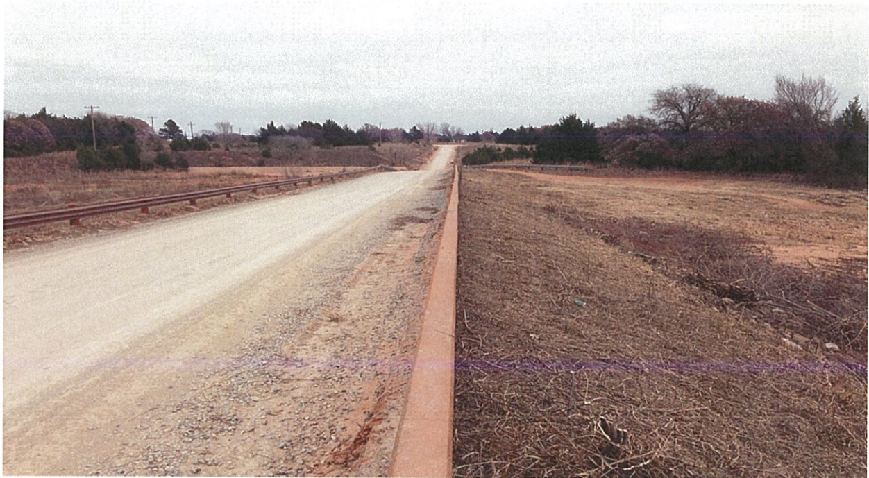
Figure 8: Crest of Dam – Photo Facing East from West Spillway
