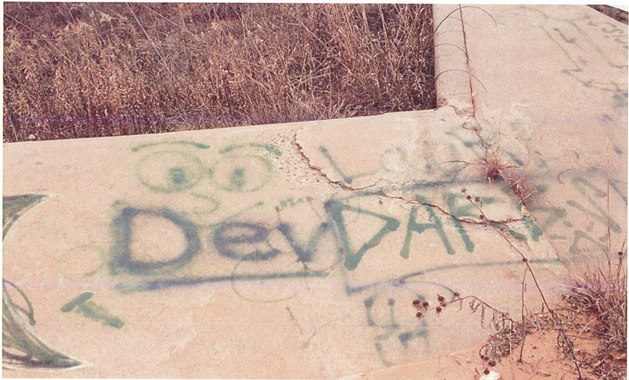
Figure 31: Emergency Spillway Abutment - Photo Facing W
